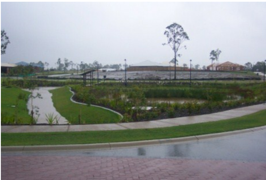
Figure SC6.4.3.9.45 Constructed wetland sediment and erosion control operation
