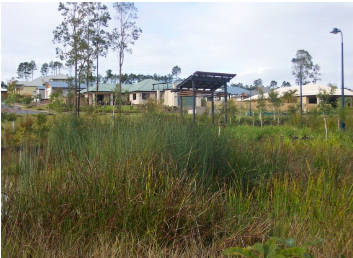
Figure SC6.4.3.9.46 Constructed wetland operational establishment
