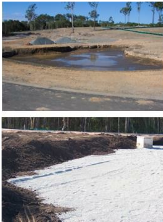
Figure SC6.4.3.9.20 Bioretention basin functional installation
