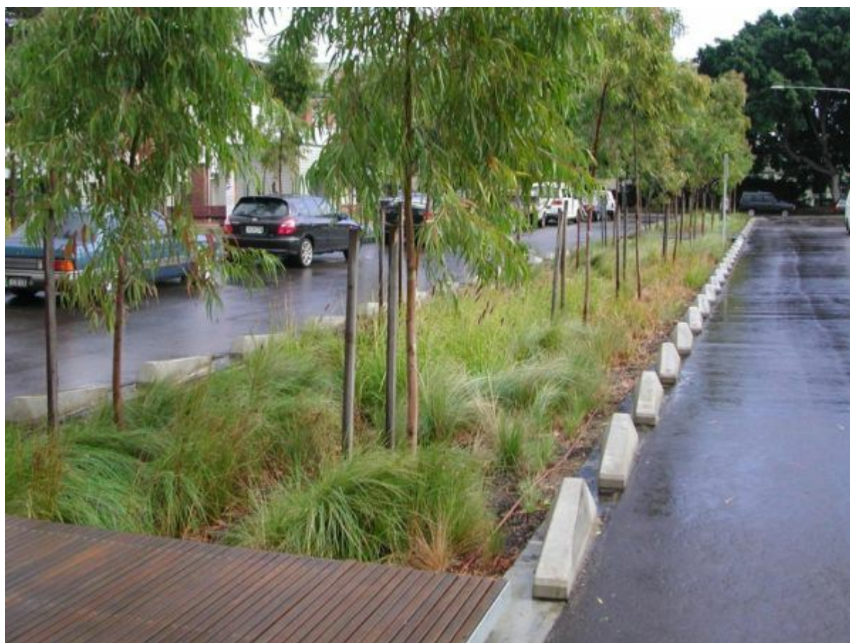
Figure SC6.4.3.9.9 Median strip bioretention applications
