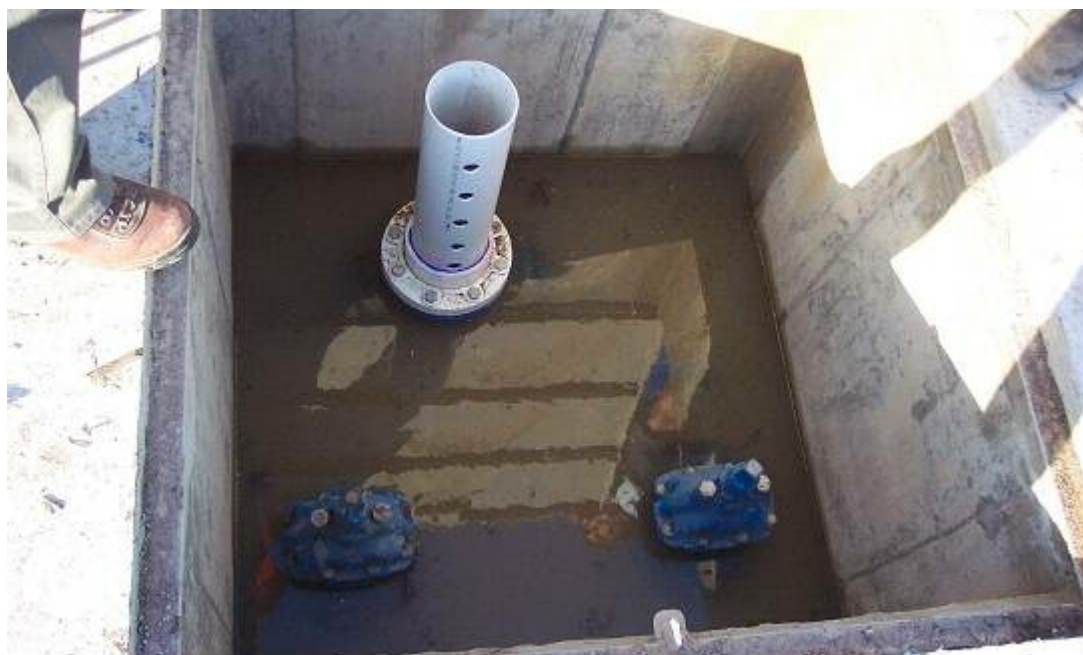
Figure SC6.4.3.9.36 Macrophyte zone outlet arrangement
