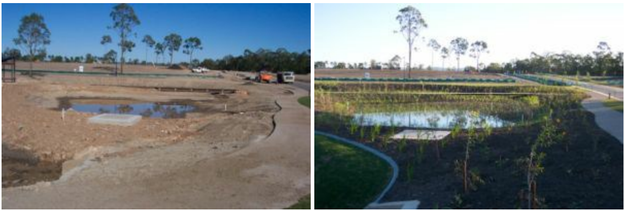
Figure SC6.4.3.9.44 depicts the functional installation of a constructed wetland
