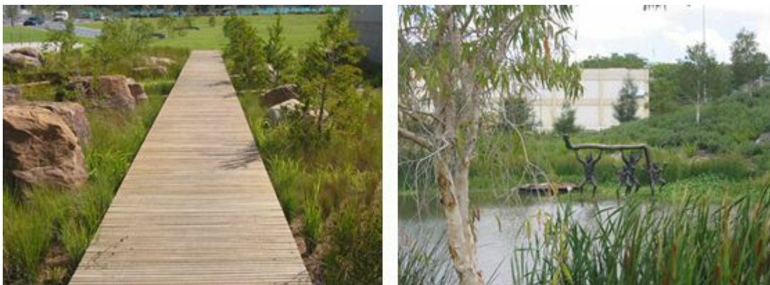
Figure SC6.4.3.9.40 Boardwalk treatment over wetland (left) and integration of urban art with wetland setting (right)
