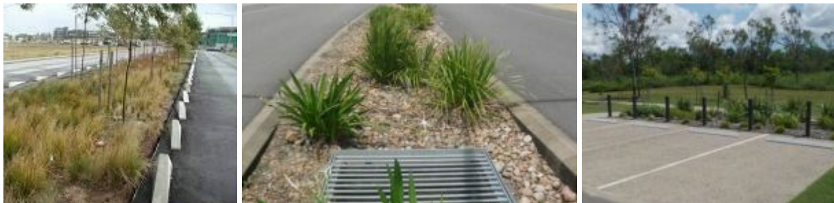
Figure SC6.4.3.9.5 Kerb arrangements with breaks and flush kerbs to distribute inflows on to bioretention swales and prevent vehicle access
