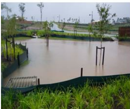
Figure SC6.4.3.9.21 Bioretention basin sediment and erosion control
