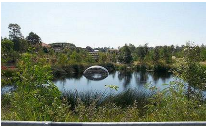
Figure SC6.4.3.9.29 Inlet zone of a constructed wetland in Brisbane
