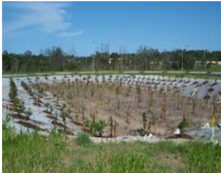
Figure SC6.4.3.9.22 Plant establishment period in bioretention basin
