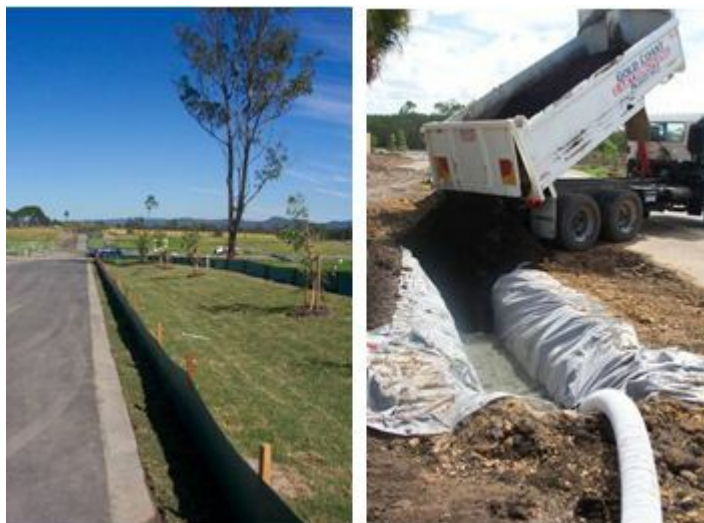
Figure SC6.4.3.9.14 Bioretention swale functional installation
