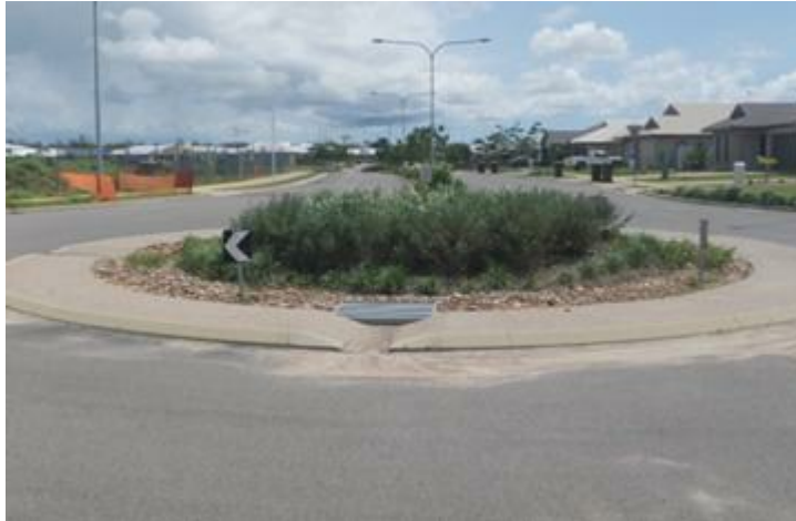
Figure SC6.4.3.9.17 Bioretention basin within roundabout at Kalynda Chase Development, Bohle Plains
