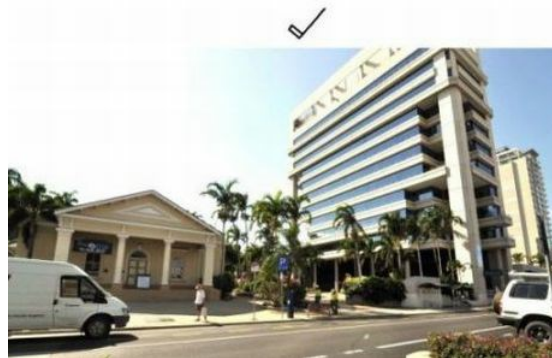
Figure SC6.3.4.10 An example of a desirable outcome – free standing tower provides a significant landscaped public piazza which acts as a separation adjacent to the heritage place
